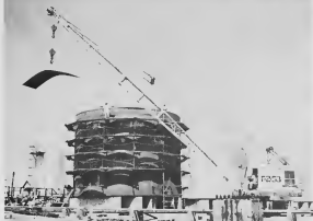
ON THE business end of a Lago crane is a sheet of steel for a nearly-completed storage tank being erected in the vicinity of tank No. 495. DEN GARA di un grua di Lago ta un plachi di stal pa un tanki casi cla cu ta wordé lamá den proximidad di tanki No. 495.
